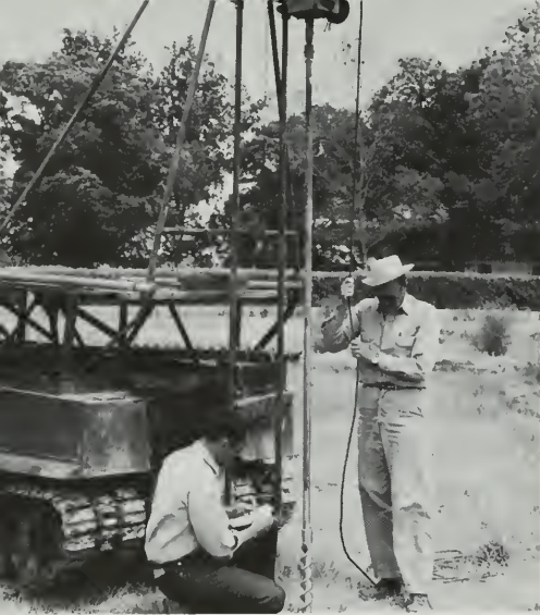
A power auger is used to get at the deeper layers of soil that influence the planning of irrigation.
